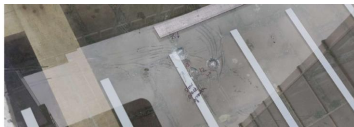
Fig. 13: Result of tests on location 5
