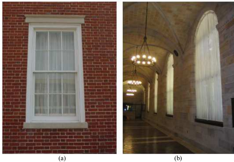
Fig. 10. Examples of application of blast curtains in residential or historical buildings (www.wincosglobal.com)
